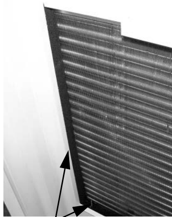
Figure 7: Air panel gasket
